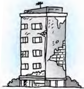
an old building
